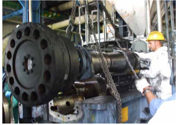
Fig. 4 - High speed shaft removal;
