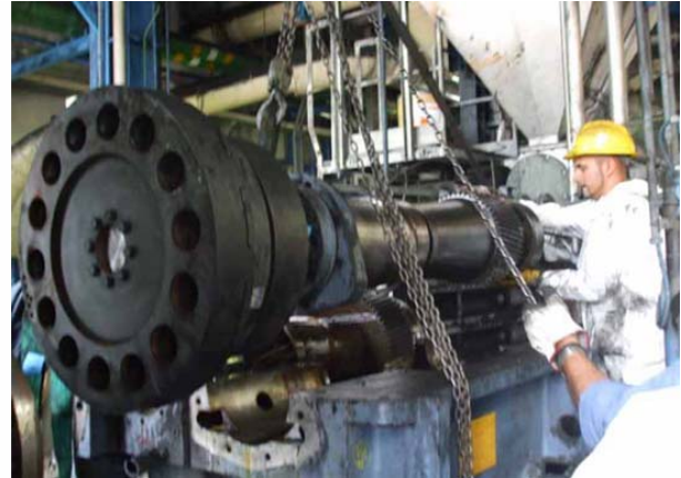
Fig. 4 - High speed shaft removal;
